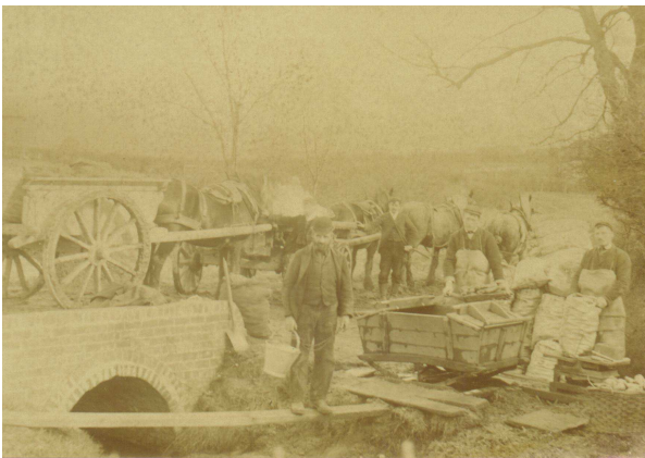
Bridge over Seggimoor Beck on Bishop Norton Road
